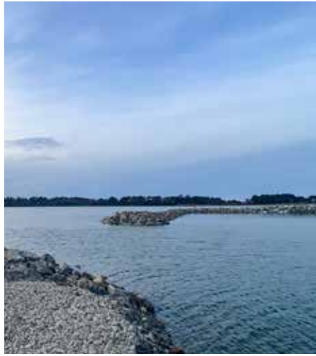
South Shore Marina's new inlet on the west side of the marina. Note the old north entrance closed off in the right of the image.
